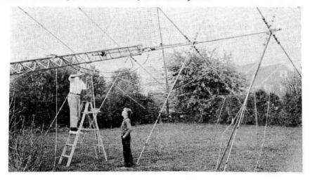
Tilt-over tower allows operator to put the finishing touches on 4 element Quad
