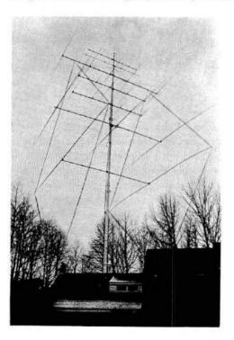
80 meter Quad dwarfs 115 foot "Christmas Tree" antenna system of K3JH. Two diamondshaped loops are used, about 50 feet on a side, plus 18 foot adjustable stubs on each element. Element spacing is 36 feet. K3JH reports good DX results with giant beam. See Chapter X for additional details and May, 1970 issue of QST magazine for full story of Quad by Joe Hertzberg, K3JH.
