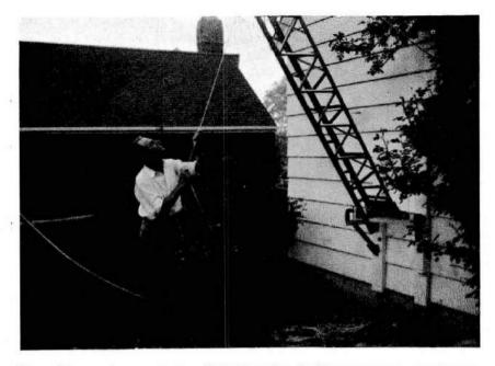
Base of tower shown on page 48 is hinged to facilitate antenna experiments. Tower base is bolted to a heavy plate hinged to two wood blocks mounted to the wall of the house. Block and tackle permits the tower to be raised easily.
