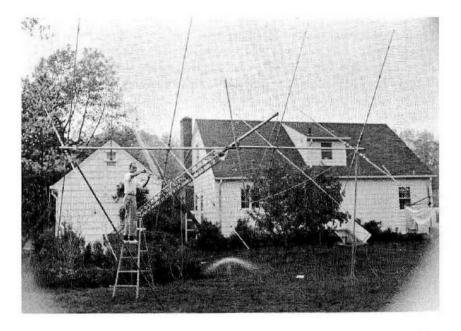
The four element Quad is ready to go up in the air. This 15 meter array employs a 22-foot boom with top and side guys. Power gain of the antenna is better than 9.4 decibels, with a front-to-back ratio of about 20 decibels.
